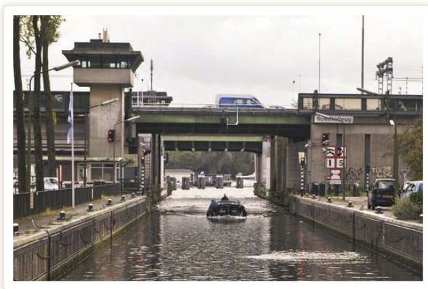
Figure 1. Example of a movable bridge (Schinkelbruggen, Amsterdam).
