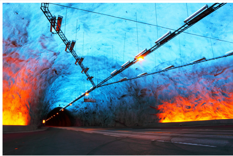
Figure 1: Daylight cave inside the Laredal-tunnel in Norway
